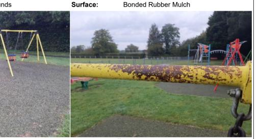
Finding: The paintwork on this item has been damaged or Action: Treat affected areas and repaint worn exposing the metal underneath which is rusting / corroding
