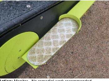
**Finding:** The tread surface does not have a 10mm high safeguard that extends around the front of the surface and at least 75% of the sides of the surface as required by BS EN 16630
