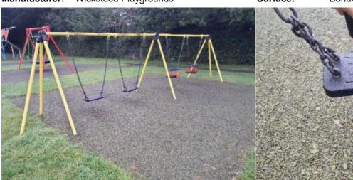
**Finding:** The seat clearance from finished surface level to the underside of the seat is too low and does not meet the requirements of BS EN 1176 Part 2 (350mm minimum clearance required)
