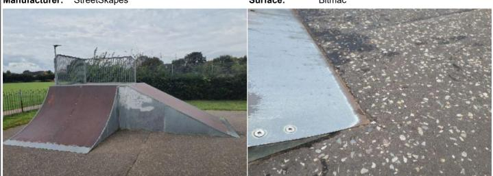
**Finding:** The kicker plate has sunk into the surface creating **Action:** Reinstate the surface to level a height differences exceeding 3mm in contravention of BS EN 14974
