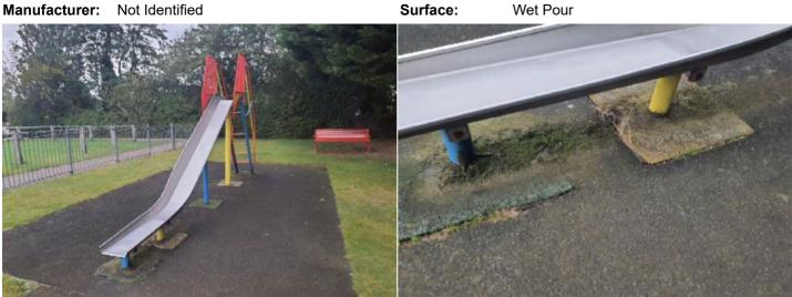
Finding: There is algae, silt or moss growth on the surface Action: Clean and treat appropriately resulting in slippery conditions
