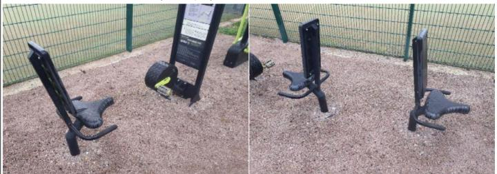
**Finding:** There are obstacles located within the movement Action: Monitor - No remedial work recommended space of the item in contravention of the requirements of BS EN 16630
