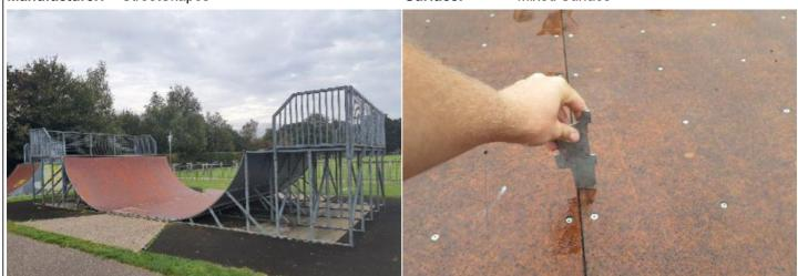
**Finding:** There is a change in the level of the rolling surface **Action:** Monitor - No remedial work recommended in excess of 3mm and the item fails the requirements of BS EN 14974 Clause 5.1.2.3
