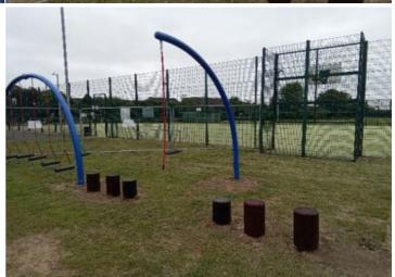
**Finding:** The item of equipment has a fall height exceeding **Action:** Refer to the designer 1.50 metres (1.70m) and grass has been provided as a safety surface, in contravention of the applicable standard
